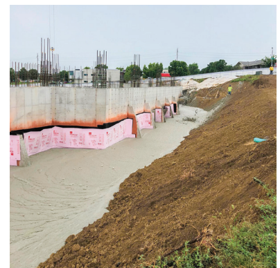
Cellular concrete placed between office building and soil nail wall
