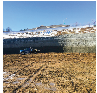
Helical soil nail wall in service prior to building construction
