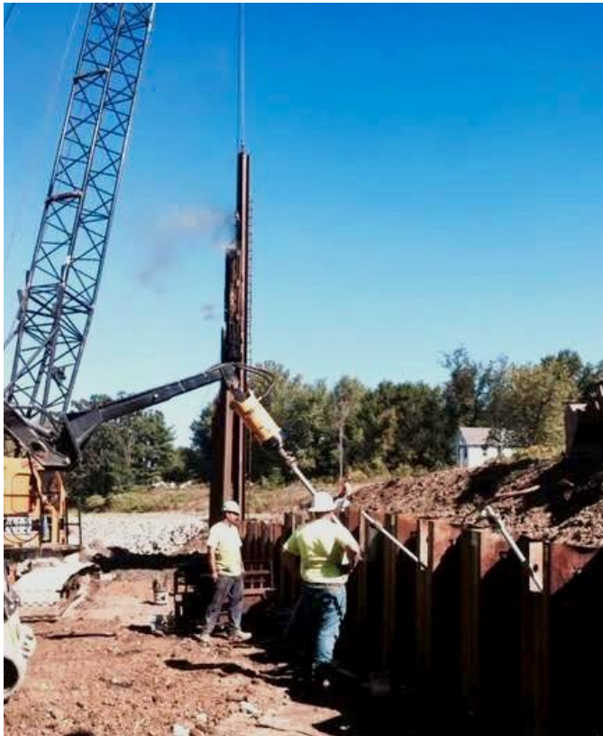
The soil bank stabilized with sheet piles and tieback anchors
