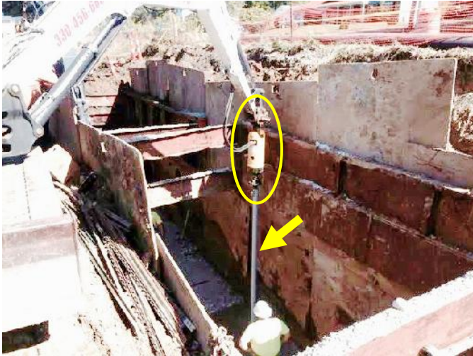
A tubular helical pile is being installed for pipe support with a Bobcat mini-excavator and a 12,000 ft-lb gear motor.
