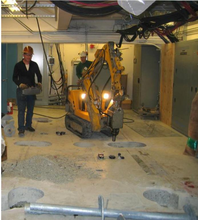
A major internet entertainment provider called McDowell Pile King, Inc. for help with slab settlement in their emergency battery room. The engineer attributed the distress to extremely heavy floor loads on the slab caused by the racks of wet cell batteries.
