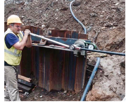
Post tensioning of tiebacks.
