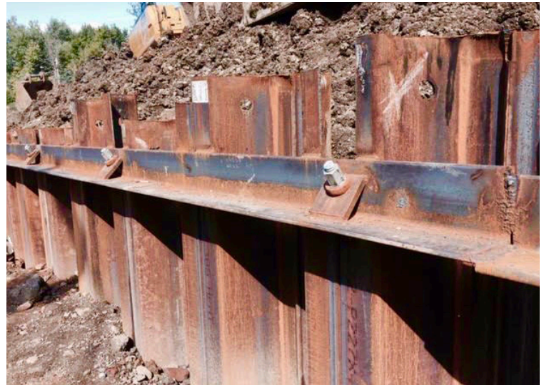
Final configuration of sheet pile wall with tiebacks.
