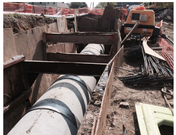
Sewer line with straps ready for backfill.
