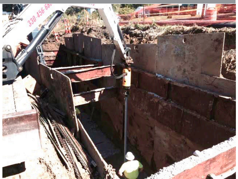
Installation of screw piling for sewer line support.
