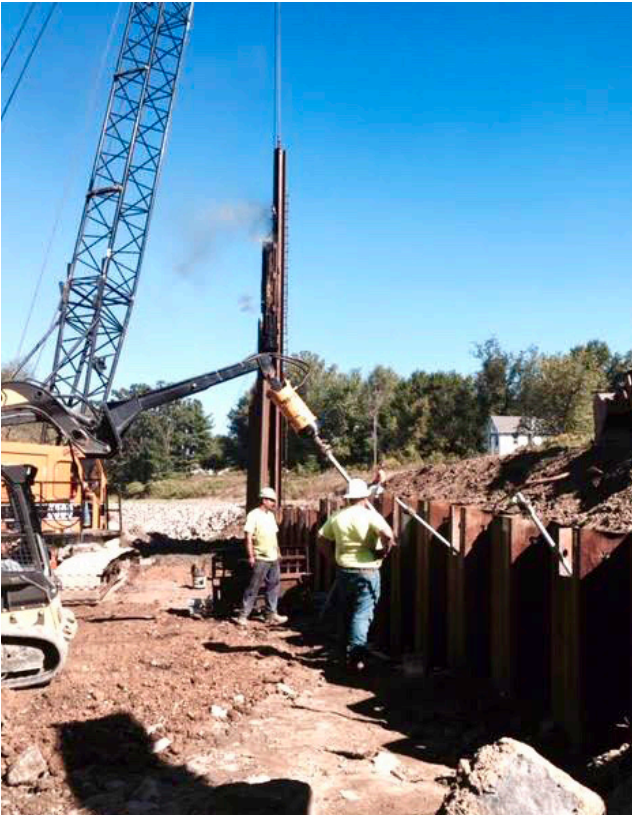
Installing sheet piles and tiebacks.
