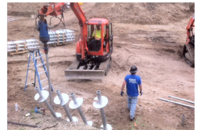
Advancing HP288 helical pile
