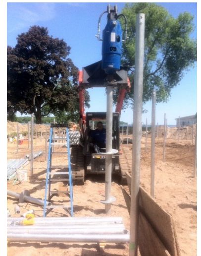
Advancing HP450 helical pile
