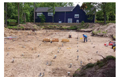
Pile installation complete
