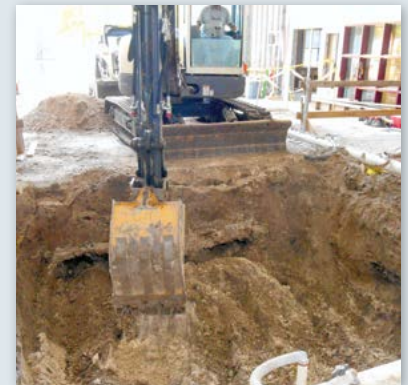
Excavation in progress
