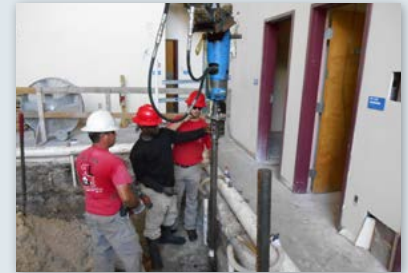
Dewatering system installed (white pipes); connecting drive head to helical pier
