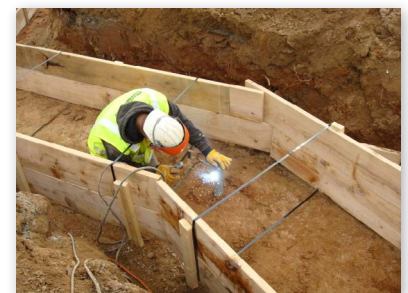
Pile caps tack-welded to shafts
