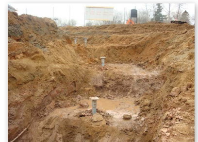
Piles in stepped grade beam
