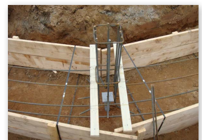
Column rebar installed
