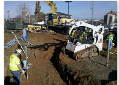
Helical piles advanced; congested working space
