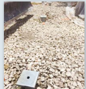
Piles installed and fitted with galvanized new construction brackets
