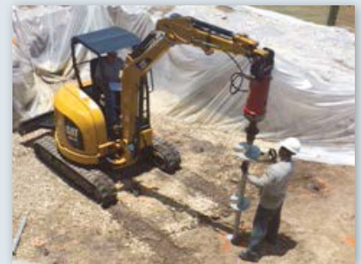
Installing helical pile lead section within pool excavation
