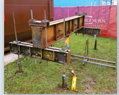
Compression load test
