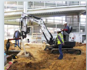
Installing helical piles within stadium
