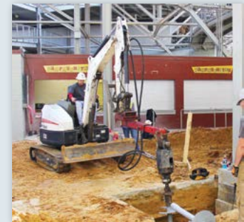
Advancing helical pile lead section
