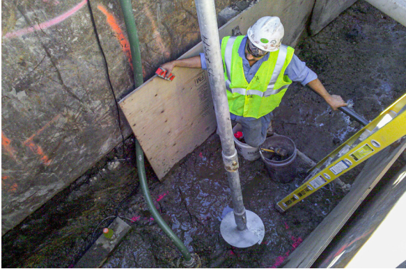
Piles advanced in shored pit for thrust block
