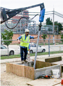
Piles installed at a batter of 6V:1H
