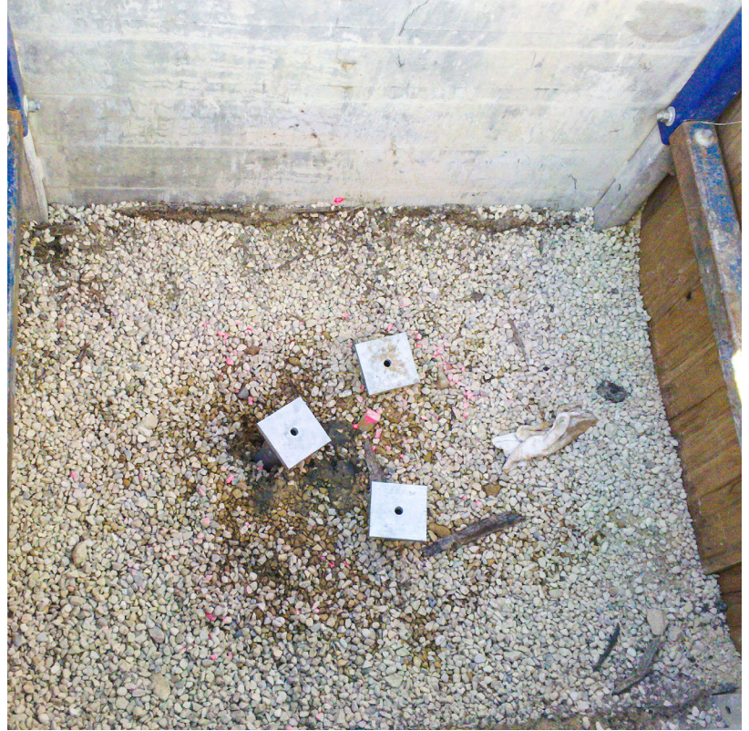
Pile installation complete for pile cap
