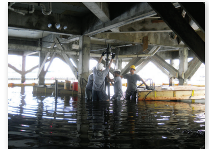
Setting handheld equipment onto helical pile
