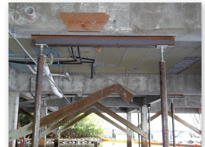
Temporary support completed
