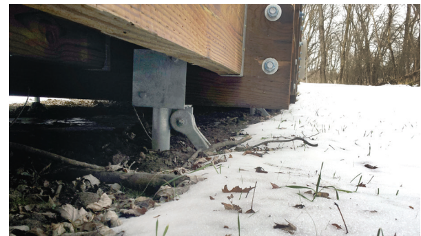
Saddle bracket with connection to battered pile
