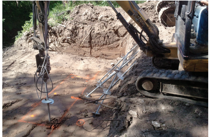
Advancing lead section at bridge abutment
