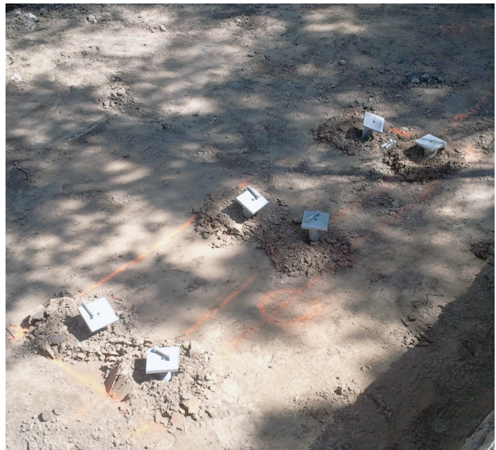
Completed pile installation at abutment
