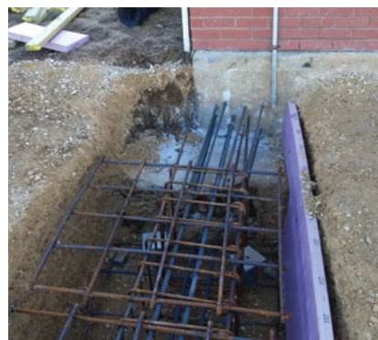
Pile cap and grade beam reinforcement installed around helical piles
