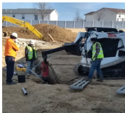
Installing helical piles with a skid steer
