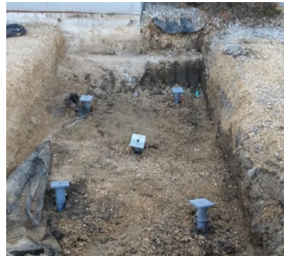
Vertical and battered helical piles within pile cap
