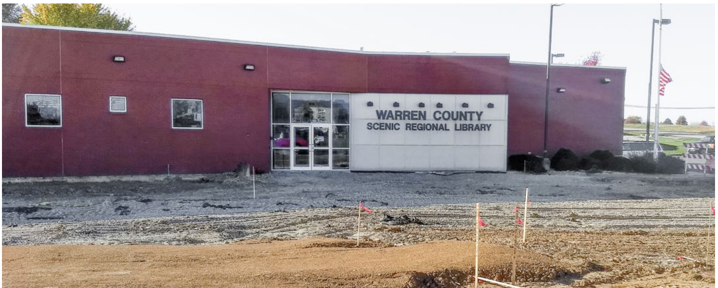
Front entrance at the start of construction
