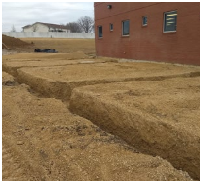
Excavations for grade beams and pile caps
