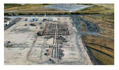
capacity calculations. Additionally, the Geotechnical Report indicated the piles may encounter early spinout due to stiff clays, and depths beyond 10ft may require pre-drilling.
