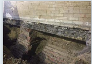
Brick wall supported by steel channels and brick piers
