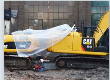
Load test using 50,000 lb. excavators as reaction
