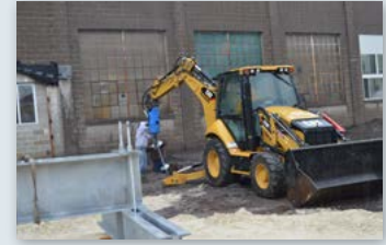
Positioning test pile lead section for installation.
