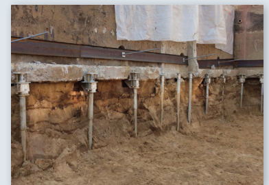
New construction/retrofit helical piles and tiebacks after excavation
