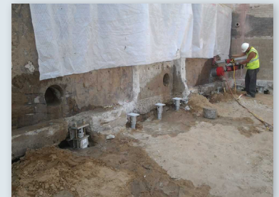
Concrete coring for helical tieback locations above new construction/retrofit helical piles
