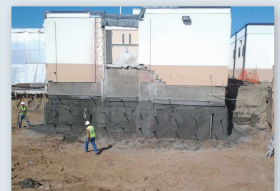
Completed shotcrete wall section
