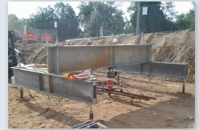
Compression load test on HP288 helical pile
