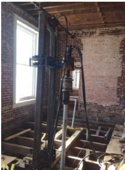
Custom mobile unit installing pile
