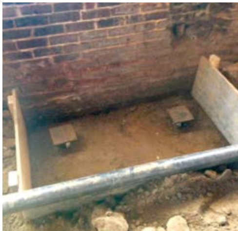
New construction caps set into new footing
