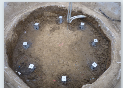
Piles cut to design elevation; brackets welded to shafts
