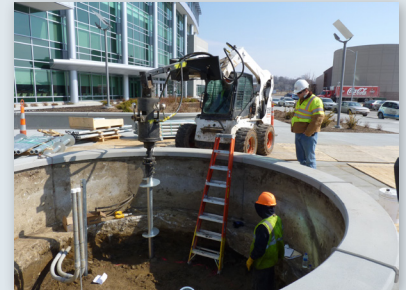
Advancing lead section
