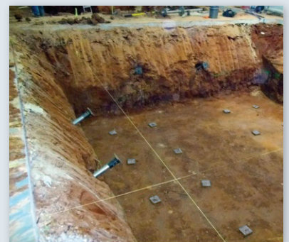
Helical piles and tiebacks successfully installed in press pit two
