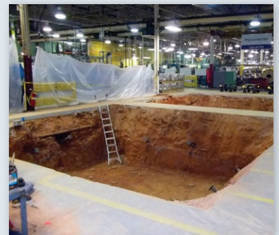
Completed press pit one (background) and press pit two post-excavation (foreground)
