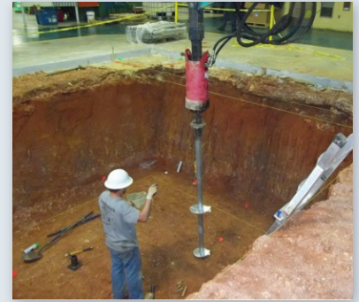
Helical piles installed to support press foundations
