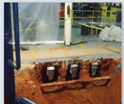
Retrofit helical piers installed to support column footings
