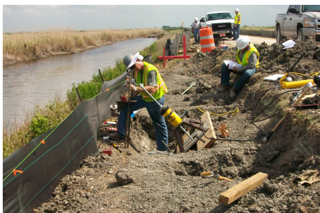
Proof testing helical tieback prior to sheet piling
