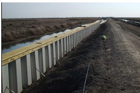
Roadway side of the seawall prior to backfill and pavement
