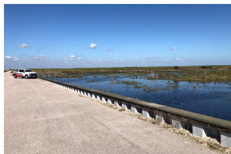
Roadway side with backfill and pavement installed
