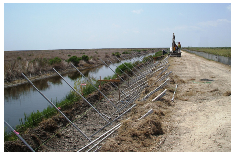
Helical tiebacks installed prior to sheet piling
