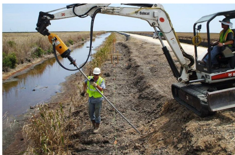
Helical tieback installation
