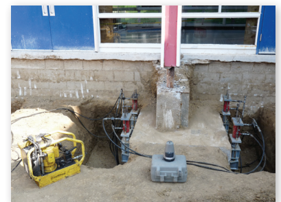
Hydraulic cylinders to apply load to the piers
