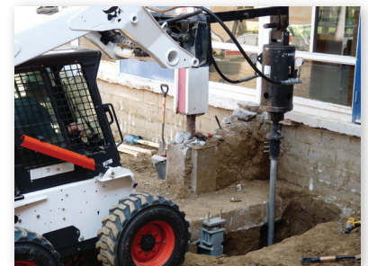
Advancing helical piers adjacent to existing column footings
