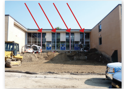
Limited working space. Four columns requiring temporary support
