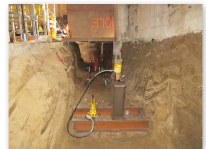
Tension test frame and equipment
