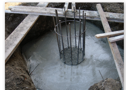
Concrete pile cap poured over helical piles
