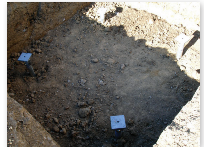
Pile installation complete
