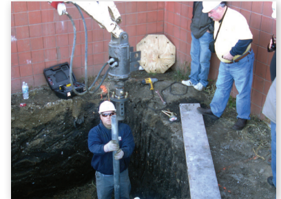
Advancing helical piles
