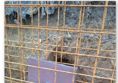
Wall reinforcement and nail head connection
