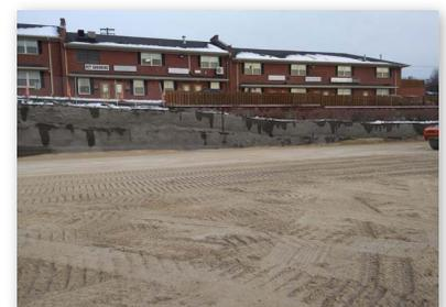
Completed helical soil nail wall
