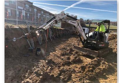
Installing helical soil nails at the north end
