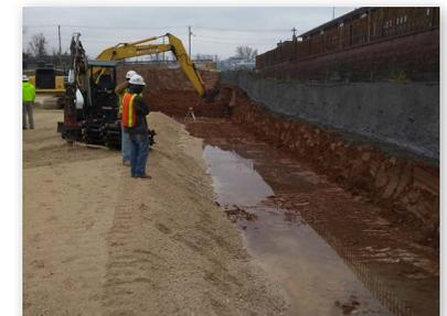
Excavation for second lift at the center wall section
