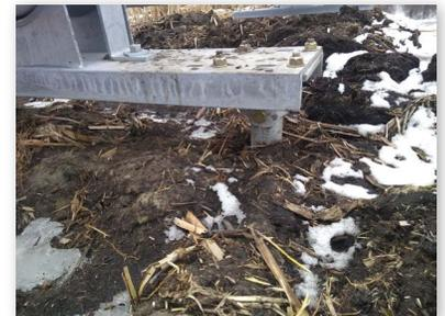
Connection of helical pile to cradle support
