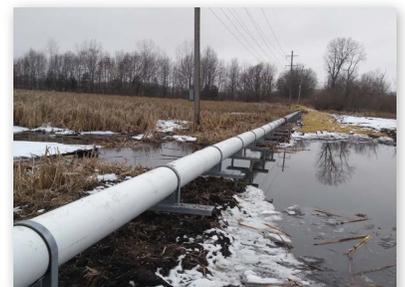
Steel cradle and helical piles support pipeline
