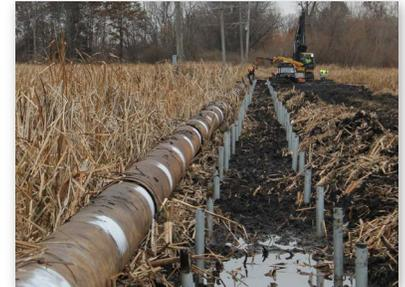
Installing helical piles adjacent to the existing pipeline and overhead utilities
