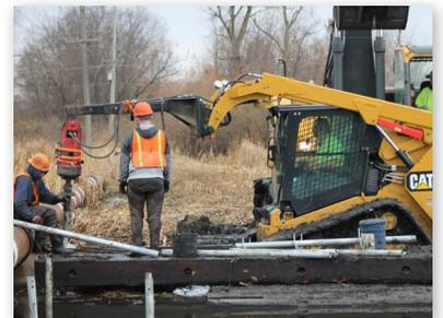
Timber matting support for the pile installation equipment
