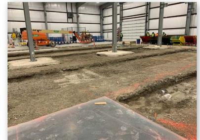
Phase 2 area prepared for pile installation around spread footings
