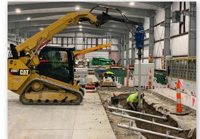
Phase 1 helical piles being installed
