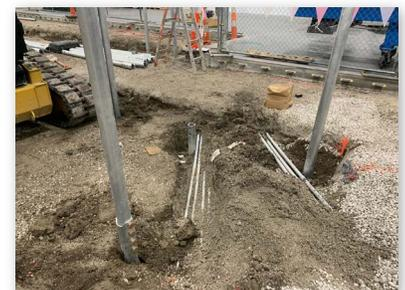
Installing helical piles around existing utilities (Phase 2)
