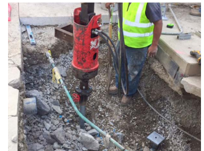
Installing around existing utilities
