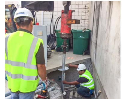
Installation of Model 288 piers near existing foundations
