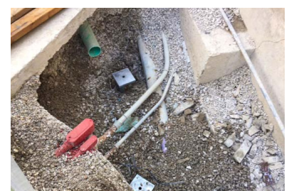
New construction brackets in place
