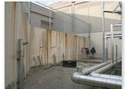
Tight access north side of wall; core-drilling 4" holes
