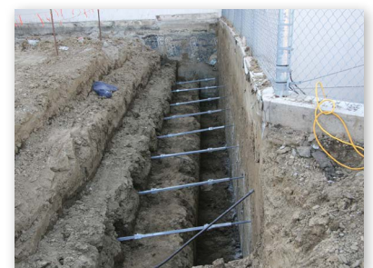
Tiebacks installed
