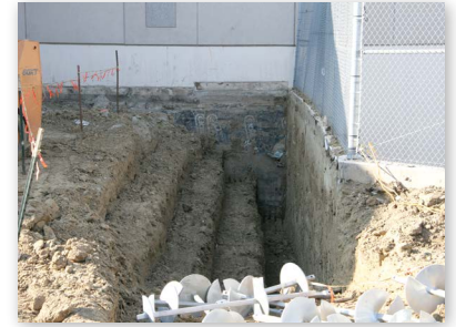
Soil excavated south side of wall
