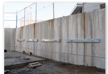
Tieback and waler installation complete
