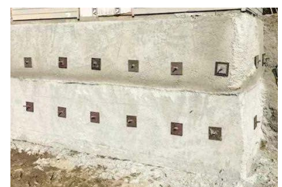
Wall completed and grouted tiebacks locked off
