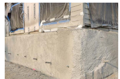
First stage shotcrete placed
