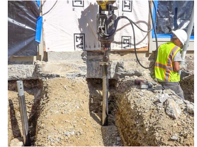
Installing retrofit helical piers
