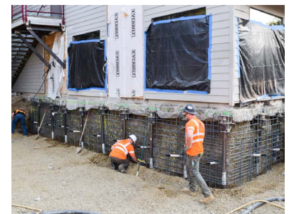
First stage shotcrete wall reinforcement installed
