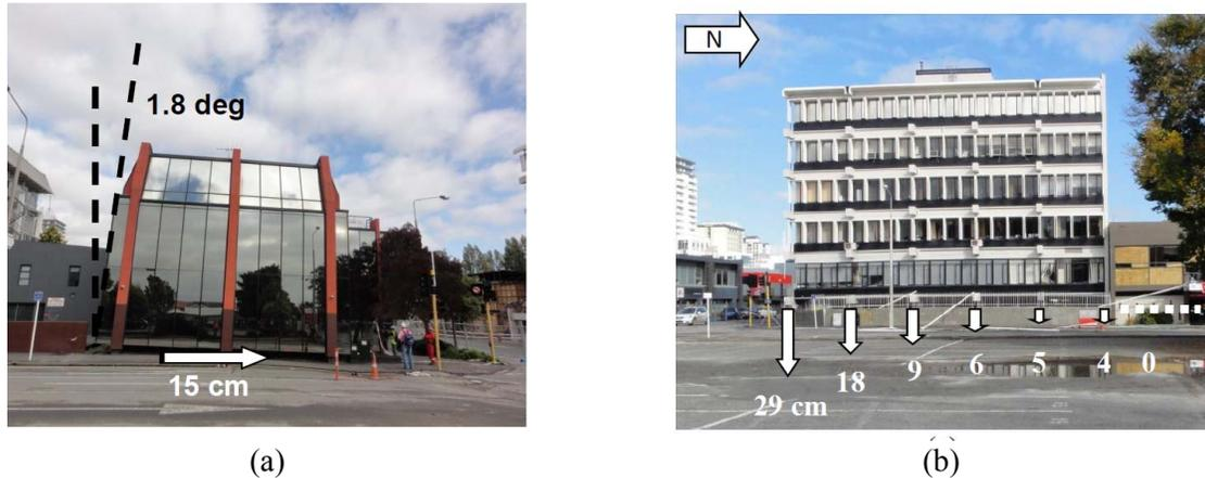
**Fig. 1. (a) Liquefaction-induced differential settlement and sliding of building of shallow-founded three-story building, (b) liquefaction-induced differential settlement in Christchurch, New Zealand (Cubrinovski et al. 2011).**
