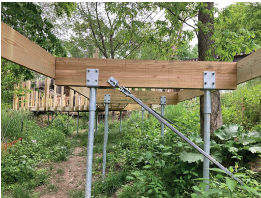
Close up of beam to pile framing.
