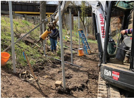
Installation of Lateral Braces.
