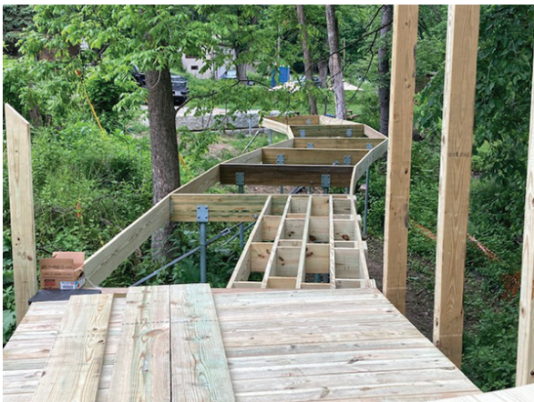
Framing of Boardwalk.
