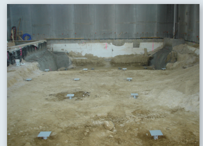
Pile installation complete
