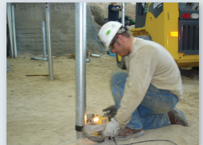
Piles cut to design elevation
