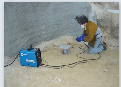
Pile caps are tack-welded
