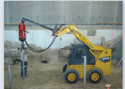
Helical piles advanced
