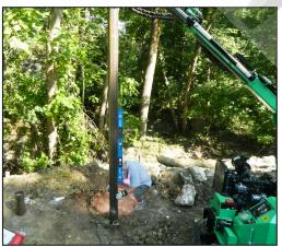
retaining wall on helical piles an effective and durable solution. The wall, being 100' long and 6' to 10' tall, depending on the section, turned out to be a challenge because of the time frame allotted for this job and the difficult area to work in, but very well worth it seeing the great looking end results.
