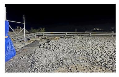
supplementary manpower to assist in the removal of the previously installed flow fill. This preparation facilitated the attachment of the necessary brackets, allowing for the subsequent installation of the helical piles.
