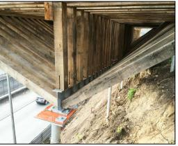
Considering the geotechnical investigation and the results of a load test, Techno Metal Post was able to propose a unique solution to support this structure in challenging conditions. Because of the specialized equipment used, the piles were installed from the top of the bank. This approach allowed traffic to run normally throughout the duration of the project.
