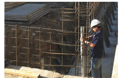
Setting pile elevations within columns and grade beams
