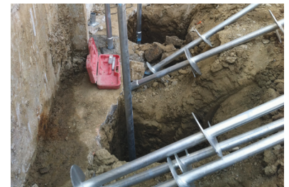
Leads and first extensions staged near installed piles
