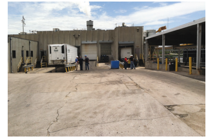
Existing loading docks
