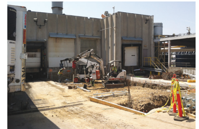
Skid-steer and mini-excavator installing helical piles
