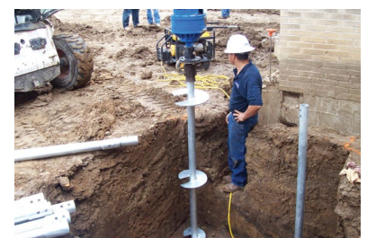
Lead section ready to advance
