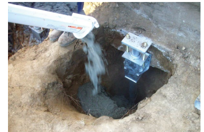
Pile and retrofit bracket installed; backfilling hole with lean concrete
