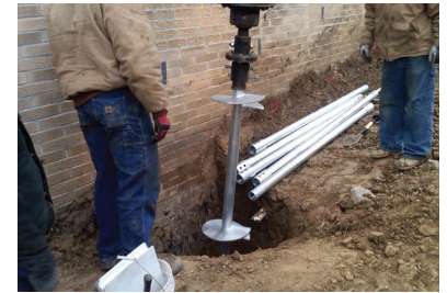
Installing retrofit helical pile
