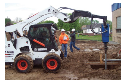
Installing new construction helical piles
