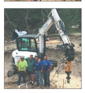
Helical Piles of NY, a division of High Rise Industries with headquarters located in Shirley, NY, recently completed installing (18) Chance Helical Piles as deep foundations for a new swimming pool in Amagansett, NY on the south side of Long Island.
