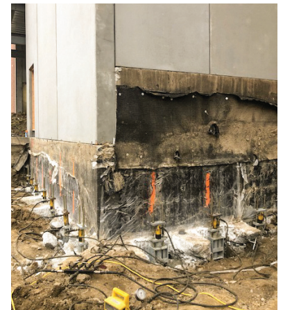
Simultaneous loading with hydraulic cylinders during lift and lock off operations
