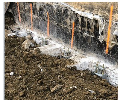
Helical piers and retrofit brackets installed
