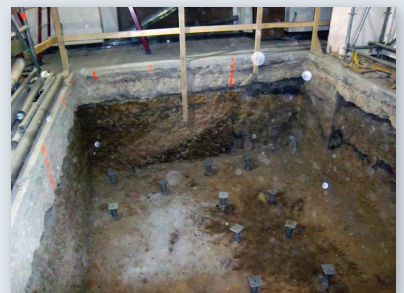
Installed piles fitted with new construction brackets
