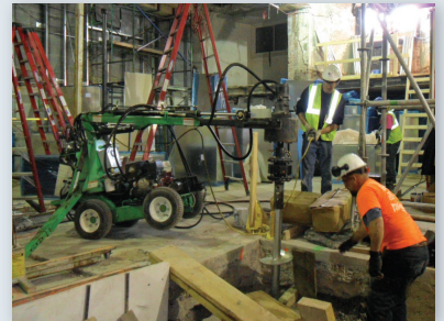
Installing HP288 lead section
