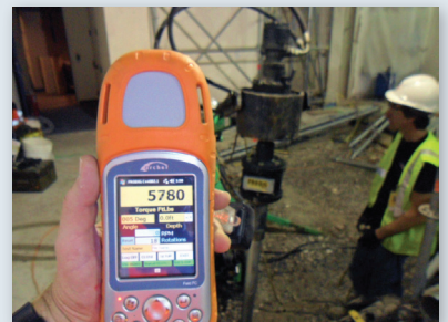
Monitoring torque during installation
