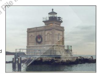
(formerly Save Huntington Lighthouse Inc.) and is an active aid to navigation with the light as the main signaling device along with the foghorn, which is maintained by the US Coast Guard. The tower height is 48 feet tall with the focal plane of the light at 42 feet above mean high water. In 1949, the Coast Guard automated the light and installed the foghorn to replace the bell.
