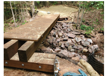
Timber abutments attached to the helical pile and anchor brackets
