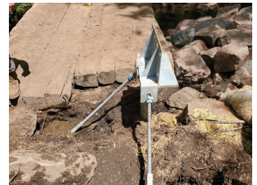
Piles, anchors, and brackets installed
