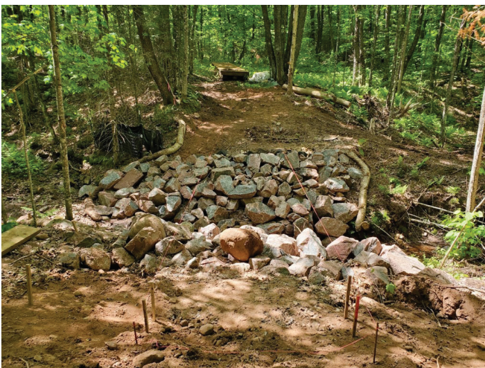
Construction preparation at one of the three bridge locations
