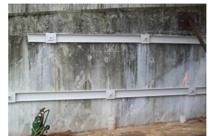
Completed tieback and waler system
