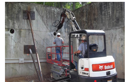
Installing top row of tiebacks; bottom waler complete
