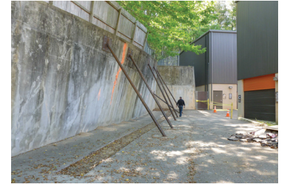
Retaining wall temporarily stabilized with steel tube bracing
