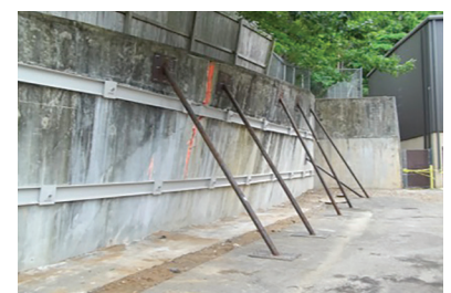
Completed tieback and waler system
