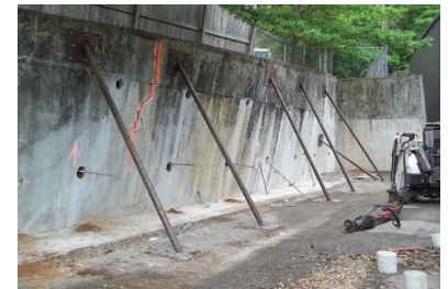
Bottom row of helical tiebacks being installed around bracing
