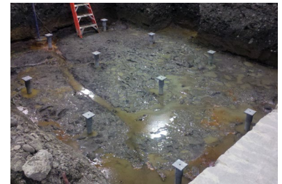
Twelve helical piles installed for each pile cap
