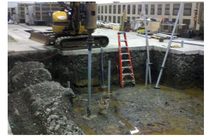
Advancing helical piles
