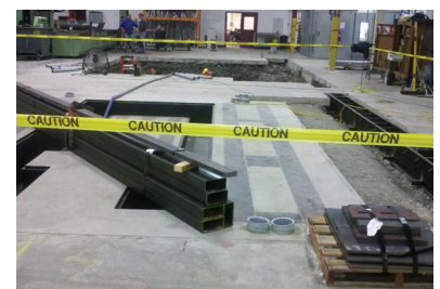
One of the two foundations near completion
