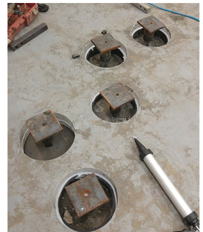
New construction pile caps in place
