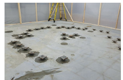
Completed Helicast piles to be embedded within the concrete foundation
