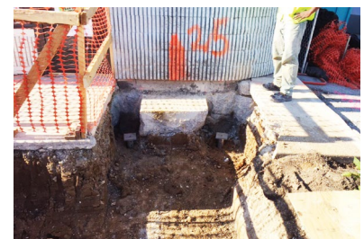
Completed piles with new construction brackets
