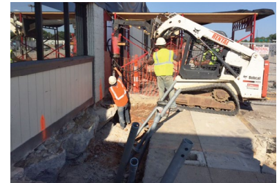
Tracked skid steer maneuvers easily within construction area
