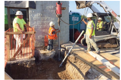
Connecting drive head to helical lead section
