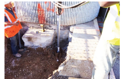
Advancing helical extension
