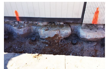
Completed piles with new construction brackets
