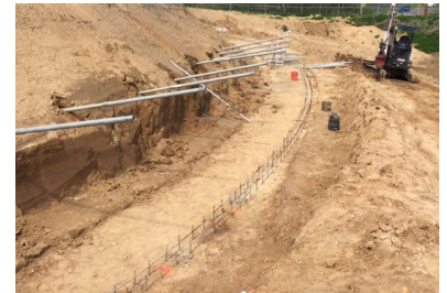
Tiebacks completed in retained soil area
