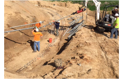
Installing HP288 helical tiebacks
