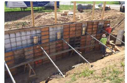
Helical tiebacks connected to wall structure
