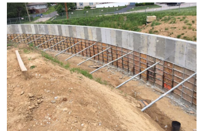
Removing forms from poured wall prior to backfill operations
