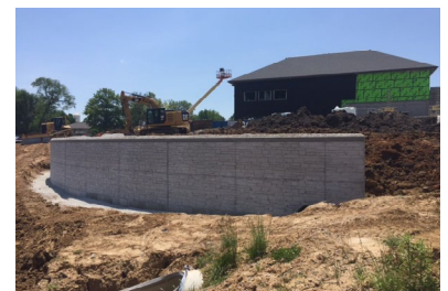
Completed and backfilled retaining wall
