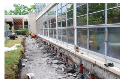
Uniform seating load applied to the piers
