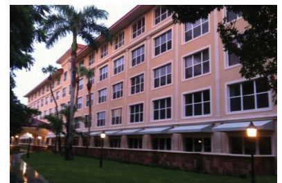
Westminster Manor after renovation
