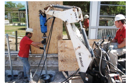
Advancing helical piers next to prepared/notched footing
