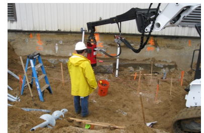
Helical piles advanced next to the existing building
