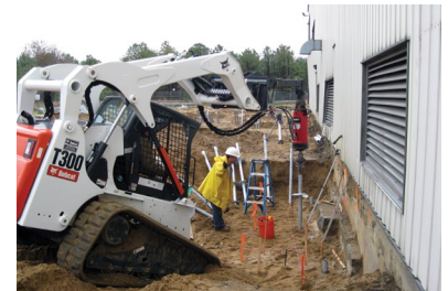
Skid steer with telescoping arm used to install helical piles
