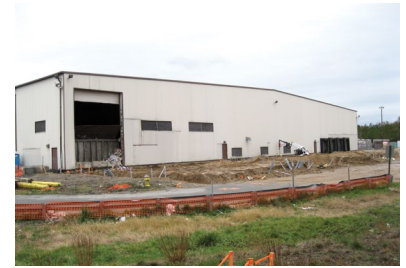
Area for the new addition
